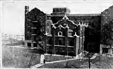
The Chapel side of the Administration Bldg.
